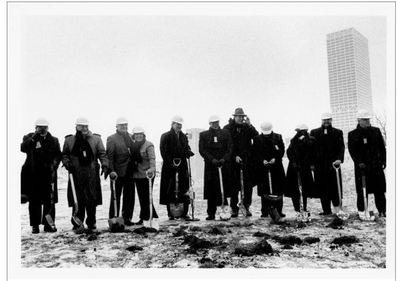
Ground-breaking for the Santiago Calatrava-designed Quadracci Pavilion, December 1997
