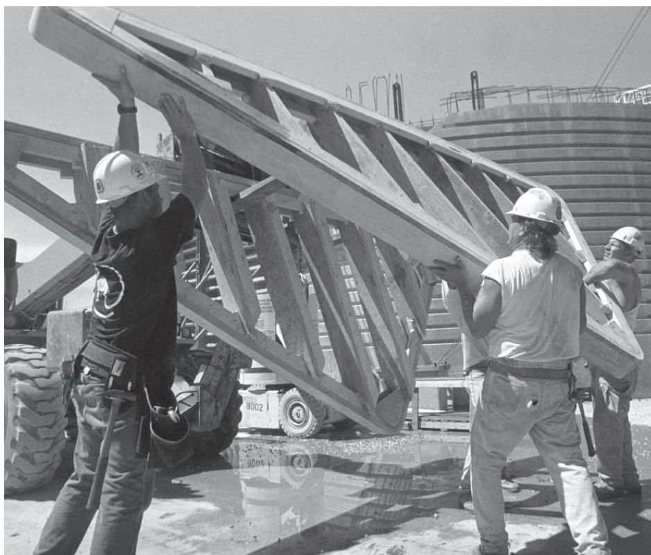
Construction of the Calatrava addition, 1999. Photo by Jim Brozek.
